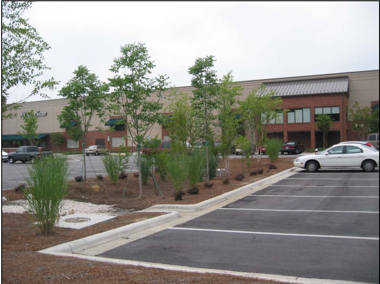
Figure 3-1. Bioretention Cell at University Mall
