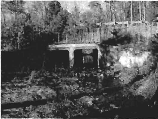
Bottomless Box Culvert (Carrboro, Turtleback crossing)
