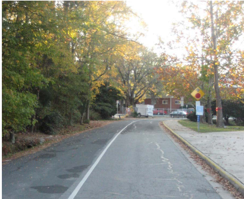
Figure 20: Pavement Markings on Shelton Street
