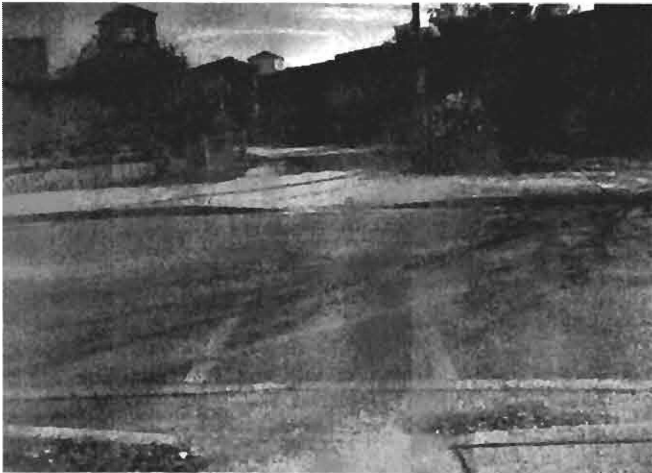
Existing crosswalks on-campus are painted onto the roadway and are fading (above). Installing high visibility thermoplastic crosswalks, as shown below in the photo rendering, will make these crossing areas safer for schoolchildren.
