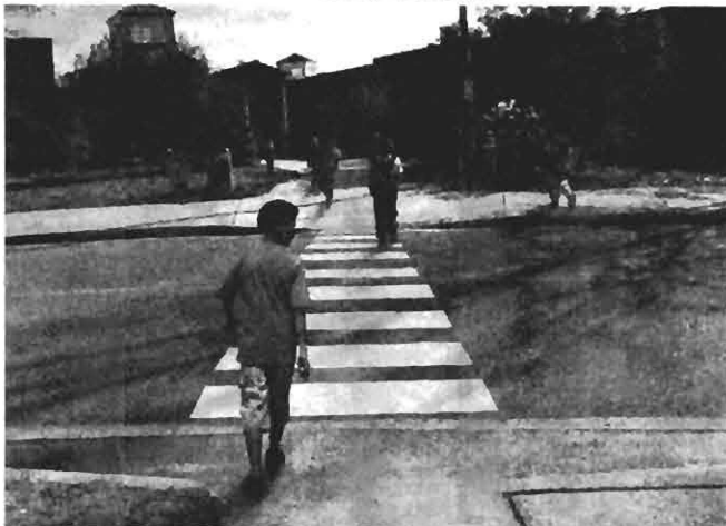
Existing crosswalks on-campus are painted onto the roadway and are fading (above). Installing high visibility thermoplastic crosswalks, as shown below in the photo rendering, will make these crossing areas safer for schoolchildren.
